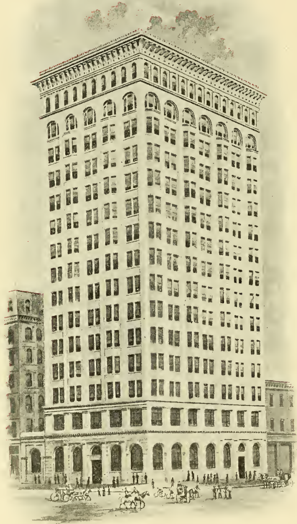
Land Title & Trust Co. Building, Philadelphia, Pa. 350 H.P. Babcock & Wilcox Boilers
